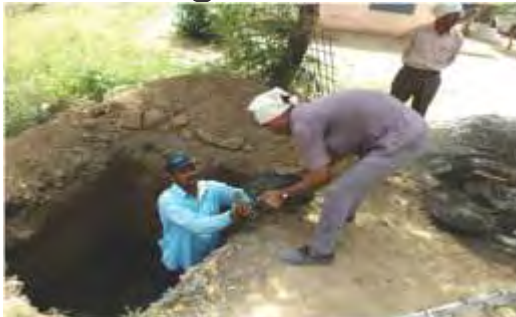
Construction Of School Gate at Vikas Vidyalaya in Nasheerabad
