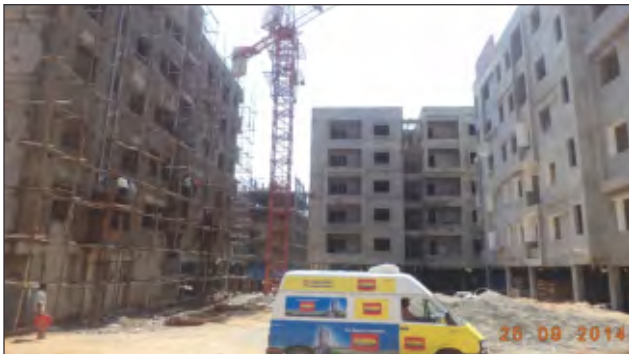
250 Flats GMR Brindavan
