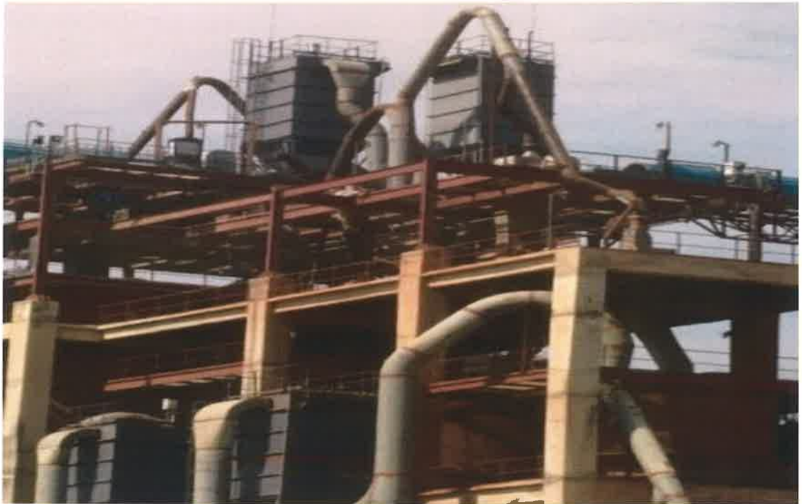
Bag Filters at all transfer points
