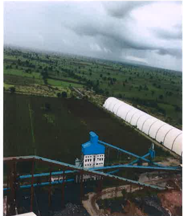
Belt Conveyors are fully covered
