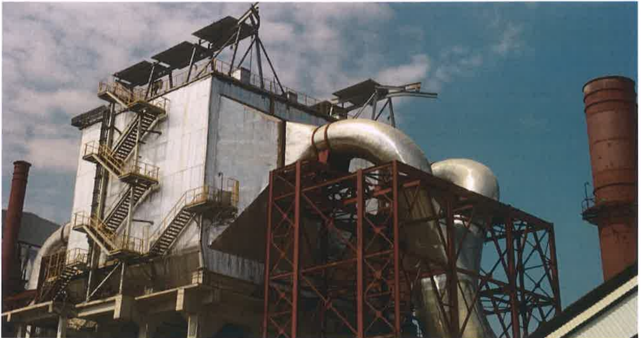
ESP for Cooler and CPP
