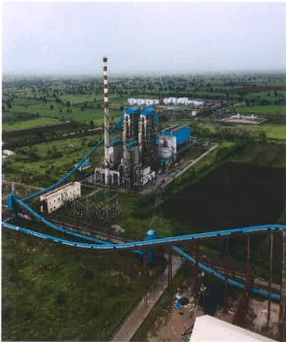
Belt Conveyors are fully covered
