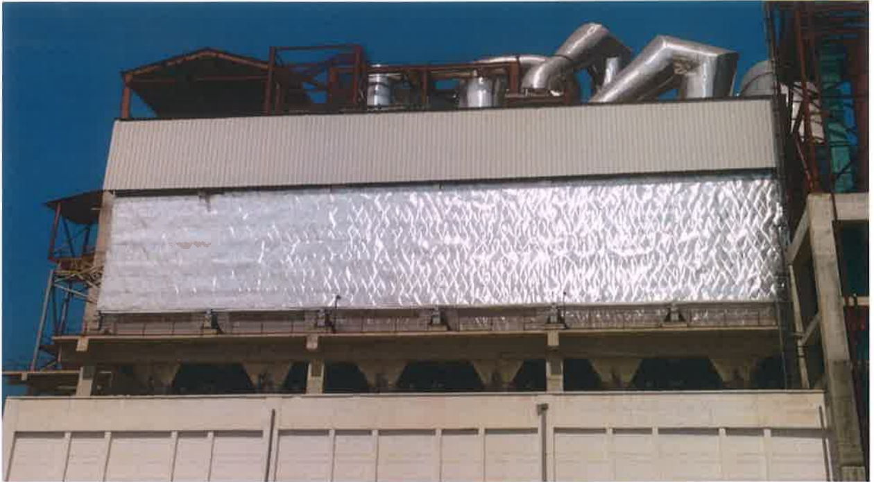
Bag House for Kiln & Raw Mill
