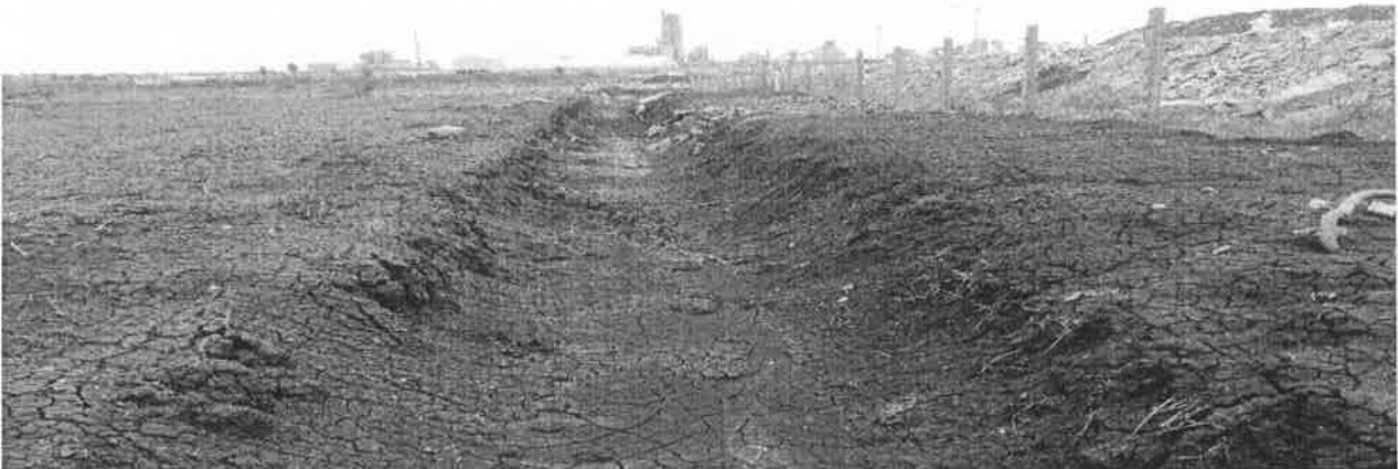
Embankment and garland drain around the pit
