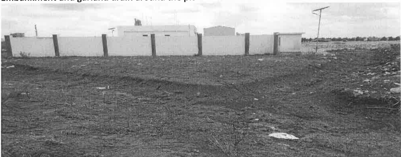
Garland drain around the pit
