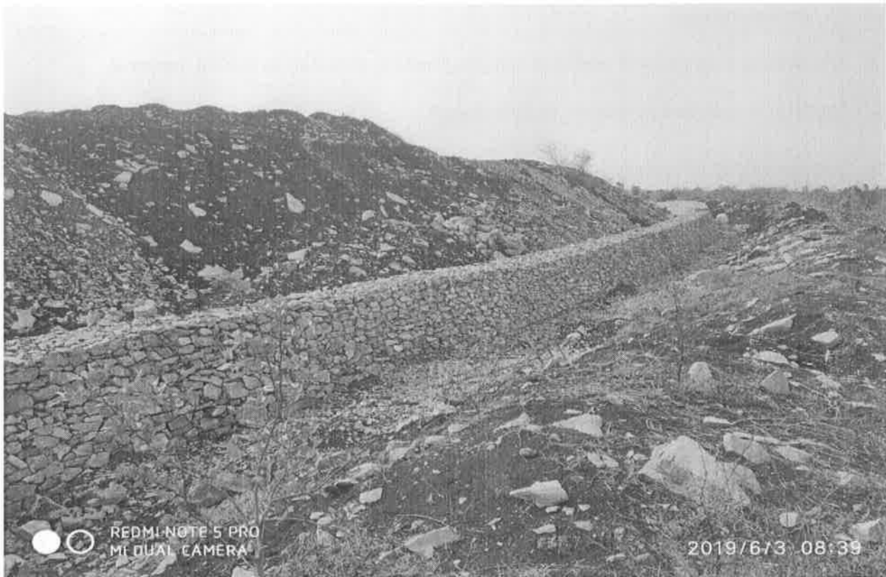
TOE WALL AT BELOW THE TOP SOIL DUMP
