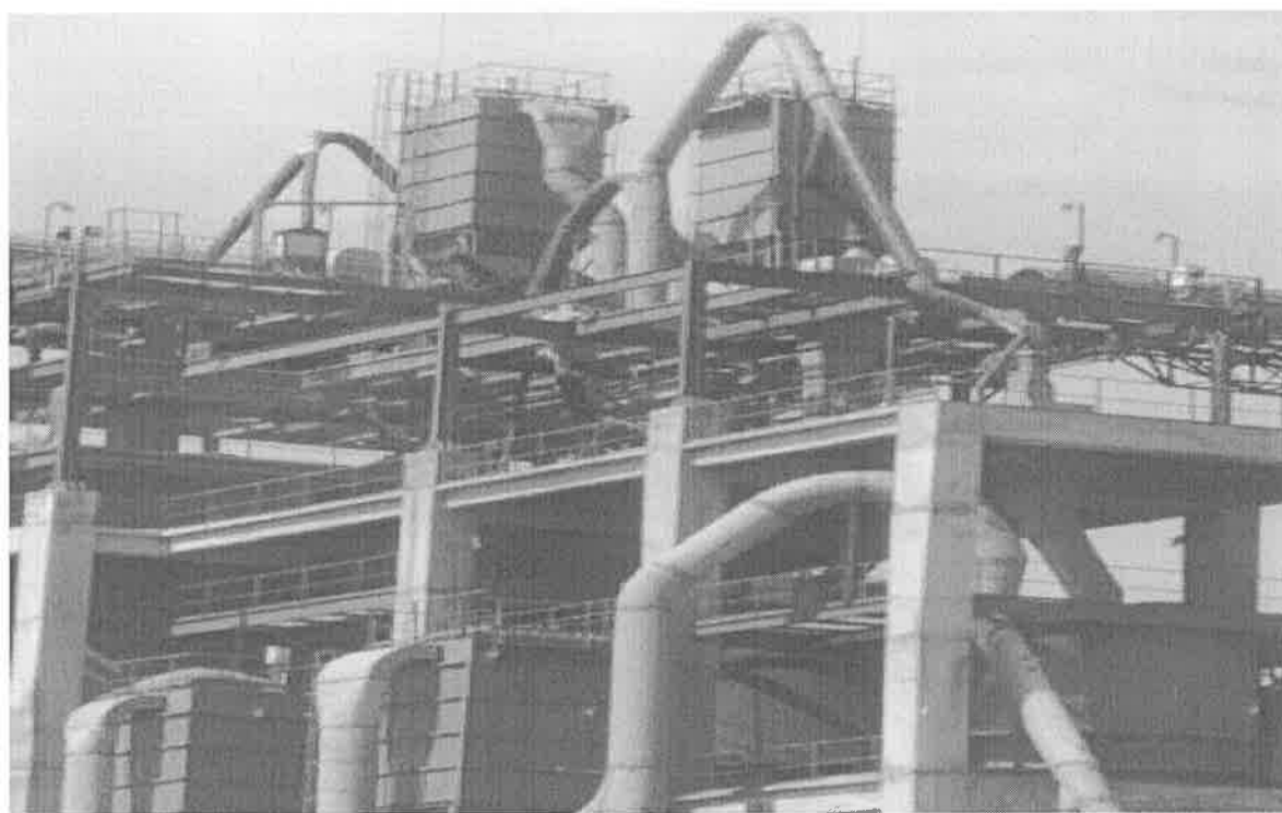
Bag Filters at all transfer points
