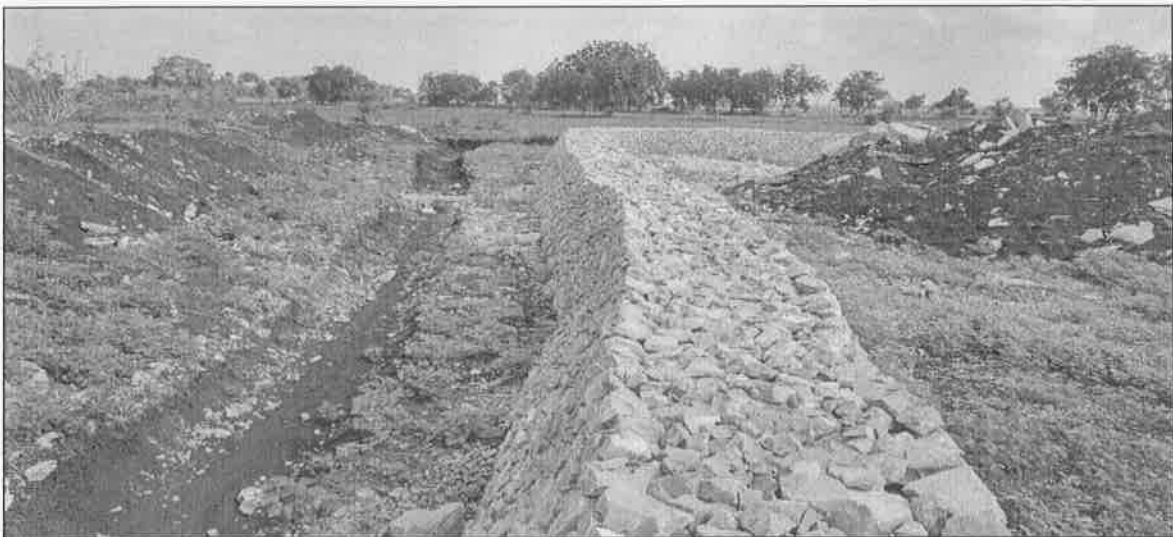
Garland Drain along the Dump Toe Wall with Random Rubble Barriers
