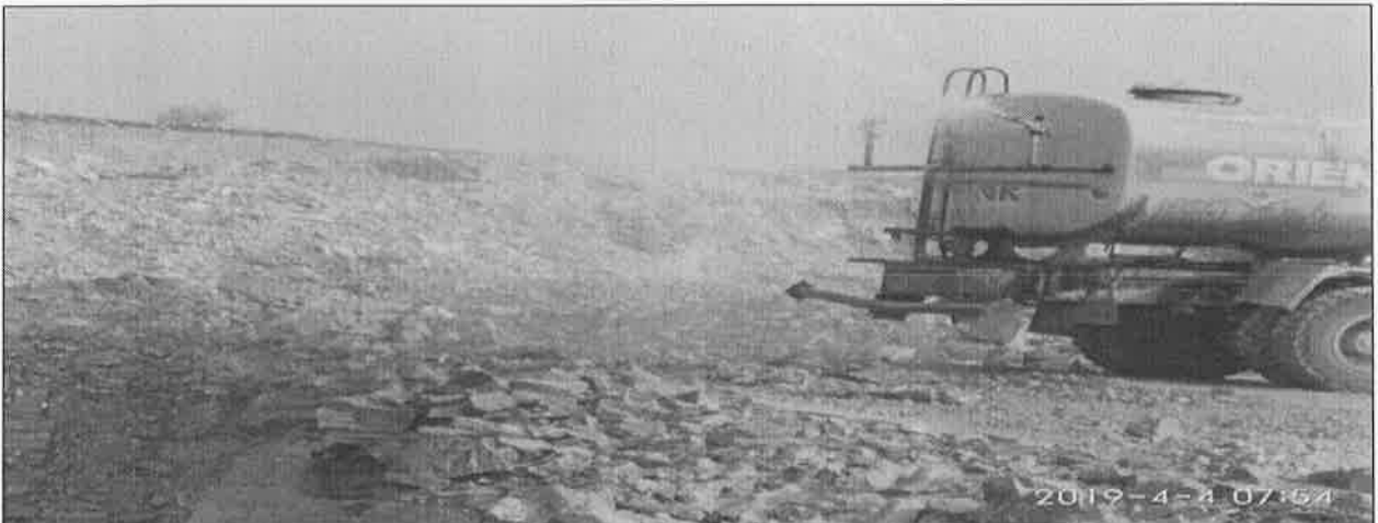
Automatic water sprinkler
