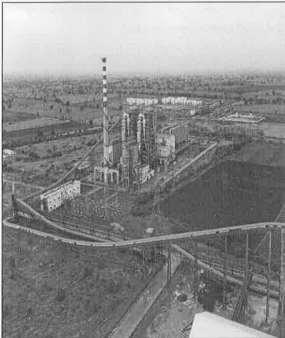
Belt Conveyors are fully covered
