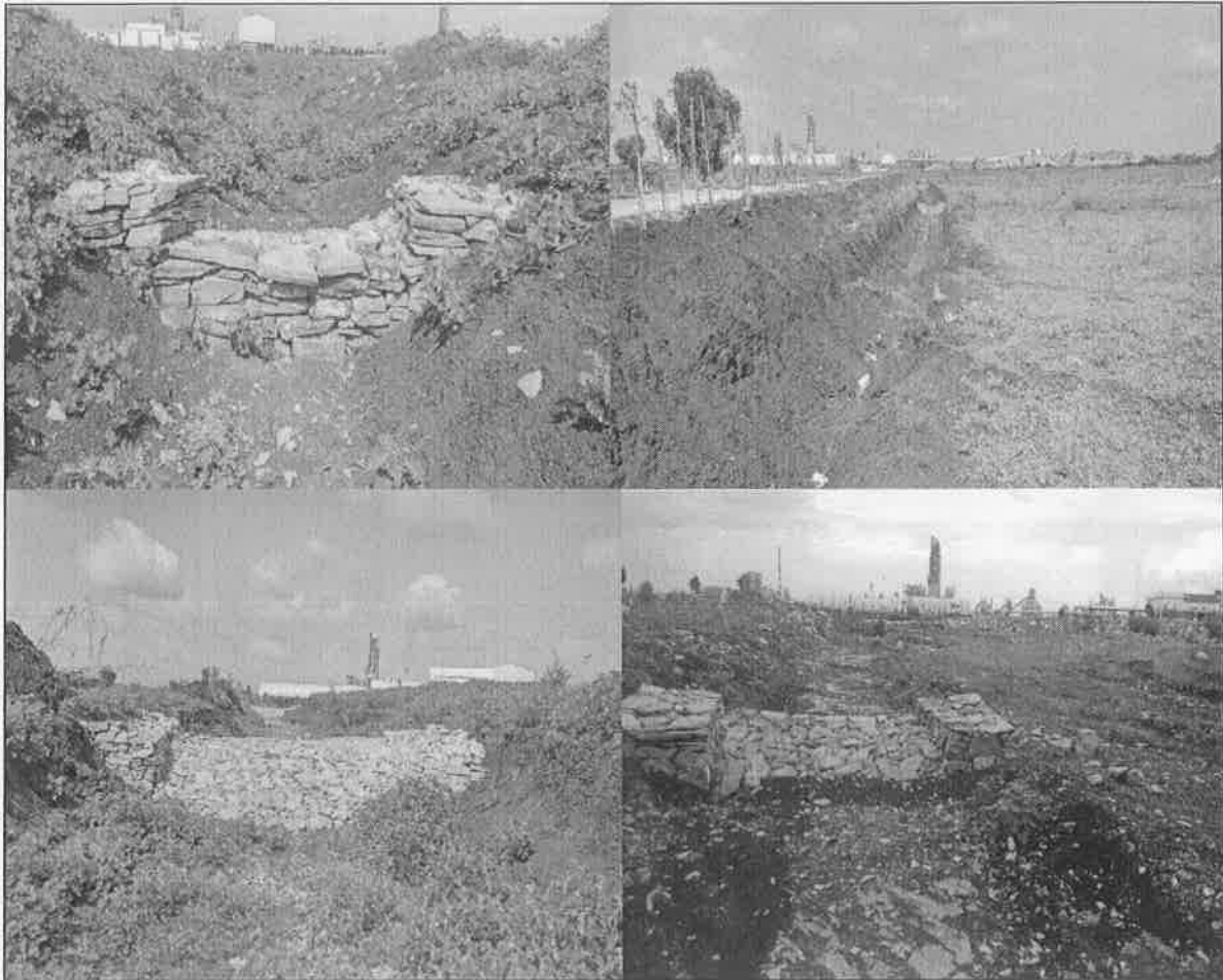
Catchment Drains with RR Dry Stone Barriers
