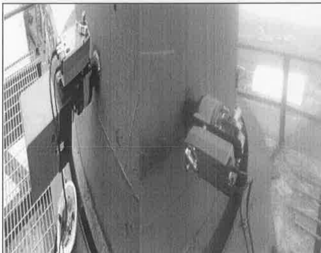
Installation of Continuous Stack emission monitoring stations for main stacks
