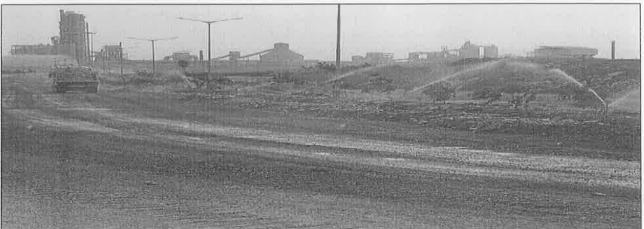
Automatic water sprinkler
