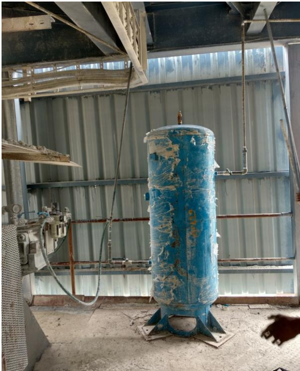
Air receiver tank with sensor at hopper to rectify air pressure drop issue
