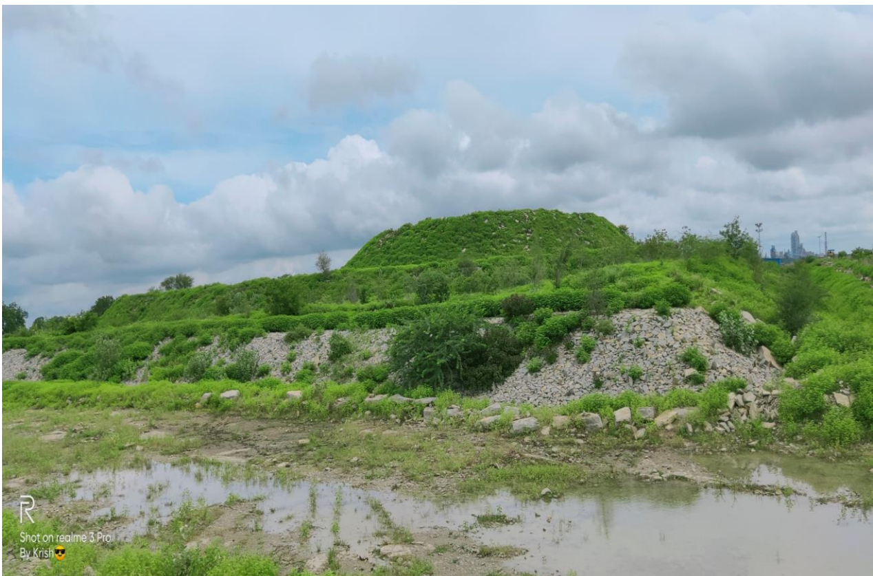
STONE PITCHING BELOW THE TOPSOIL DUMP
