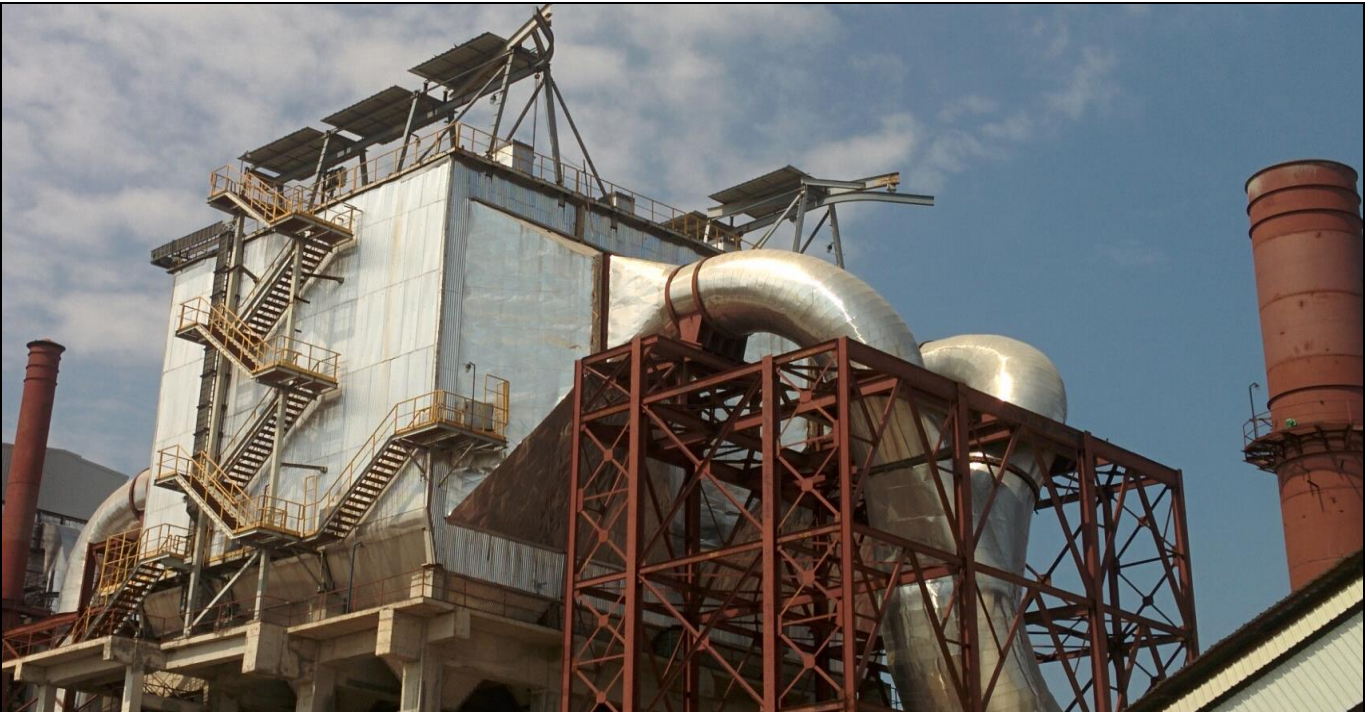
ESP for Cooler and CPP
