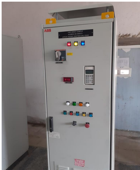
Variable Frequency Drive in 111AF060 Apron feeder
