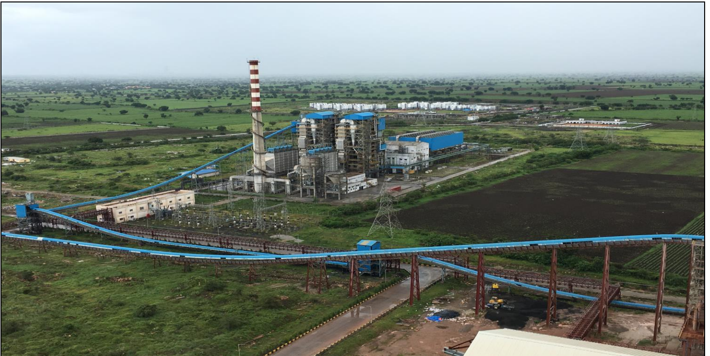
Belt Conveyors are fully covered
