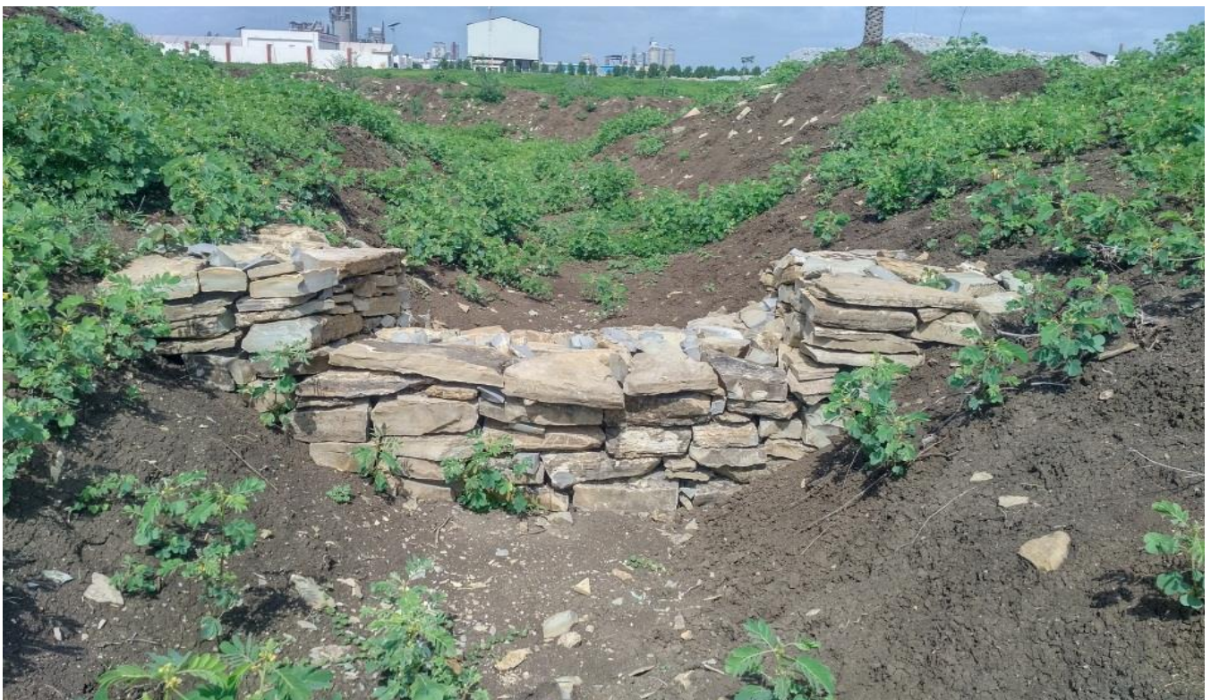
CATCHMENT/GARLAND DRAINS WITH RR DRY STONE BARRIERS
