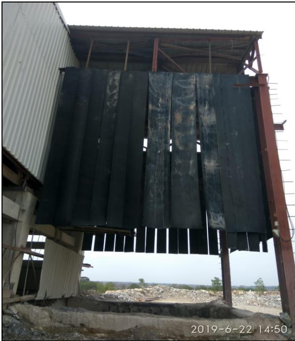
Water sprinkling & rubber Curtains @ Limestone Hopper
