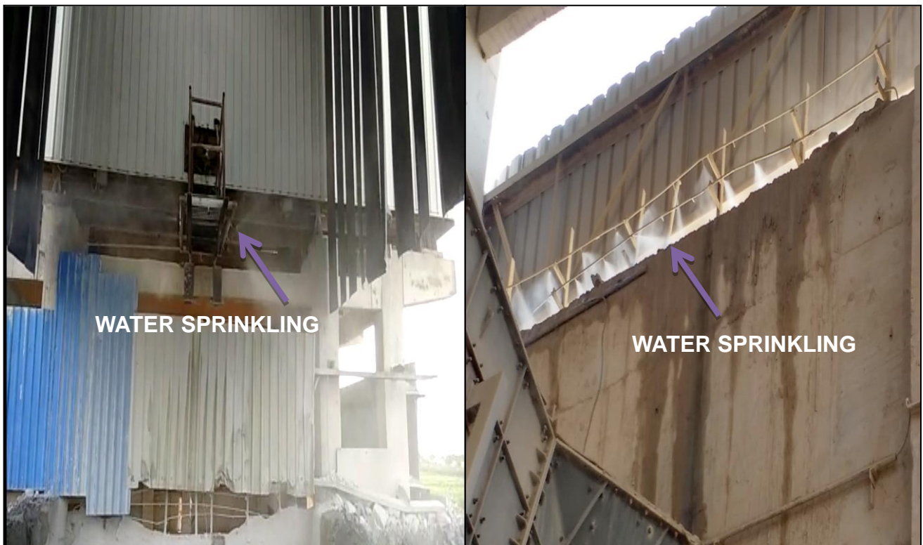
Dust Control System at Lime stone Crusher
