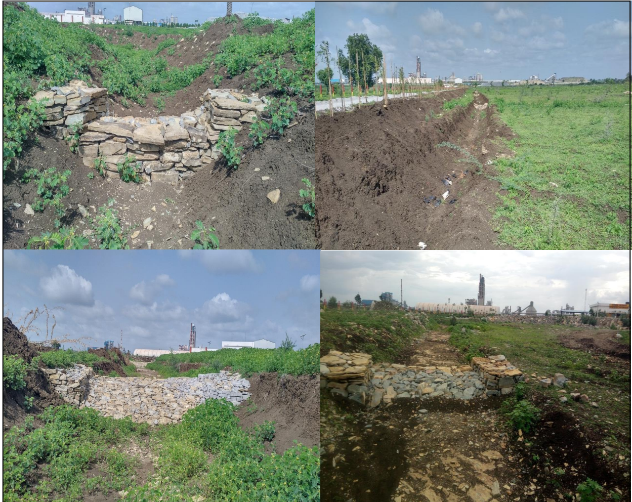
Catchment Drains with RR Dry Stone Barriers
