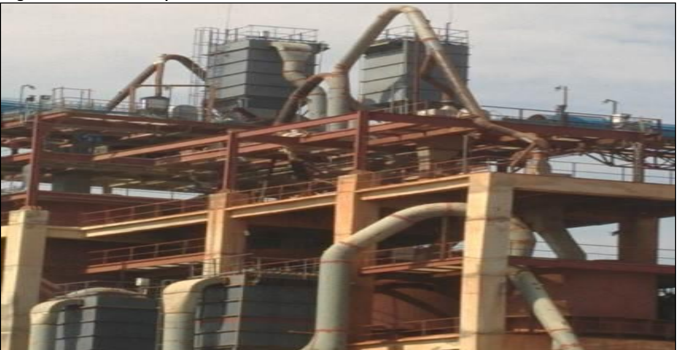
Bag Filters at all transfer points
