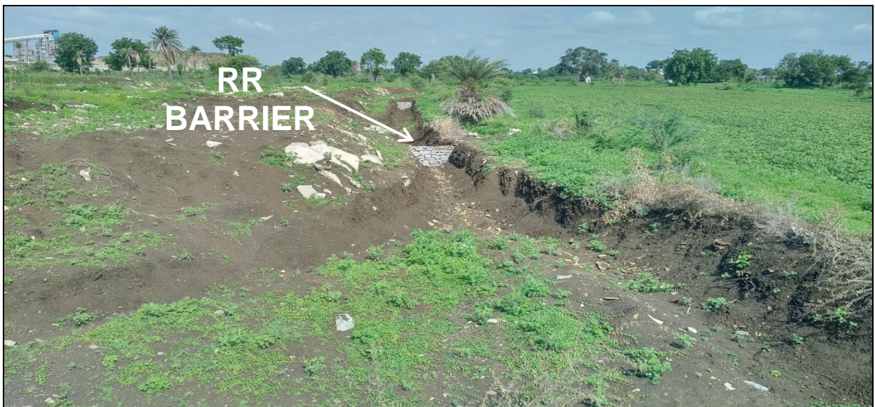
Garland drain with RR barrier
