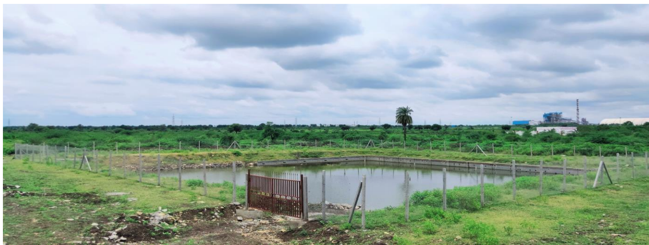
RAINWATER HARVESTING PIT cum SETTLING TANK
