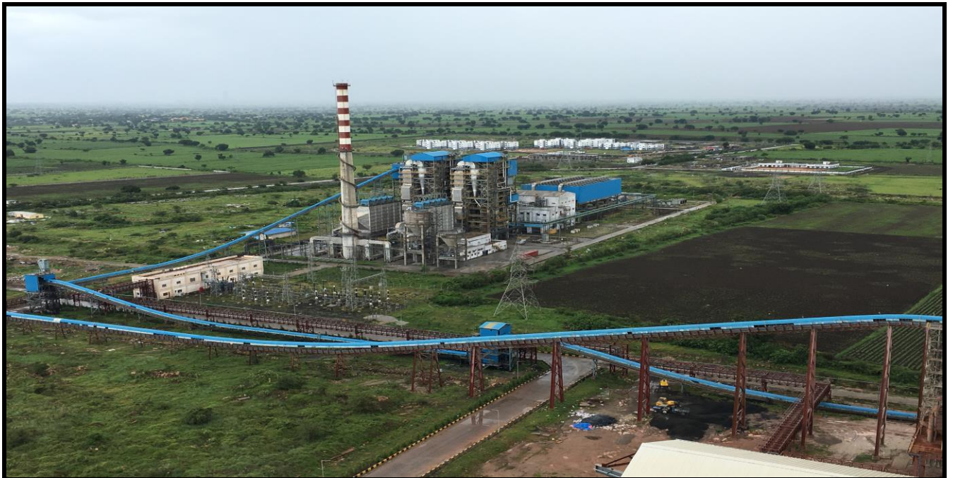
Belt Conveyors are fully covered
