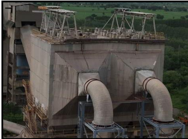
ESP for Cooler and CPP
