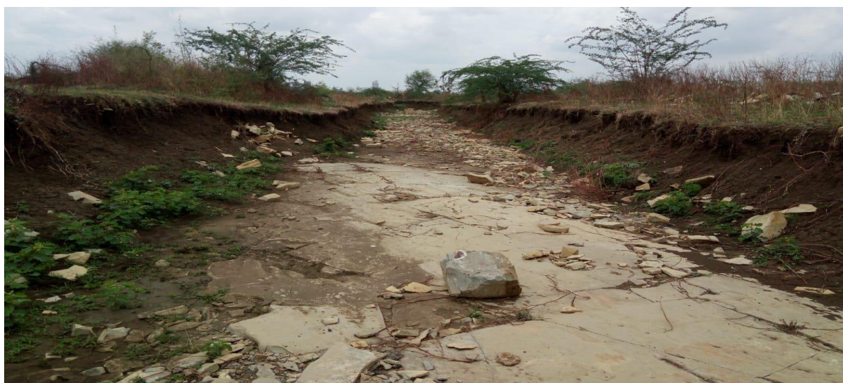
GARLAND DRAIN ALONG THE TOPSOIL DUMP TOE WALL WITH RANDOM RUBBLE BARRIERS
