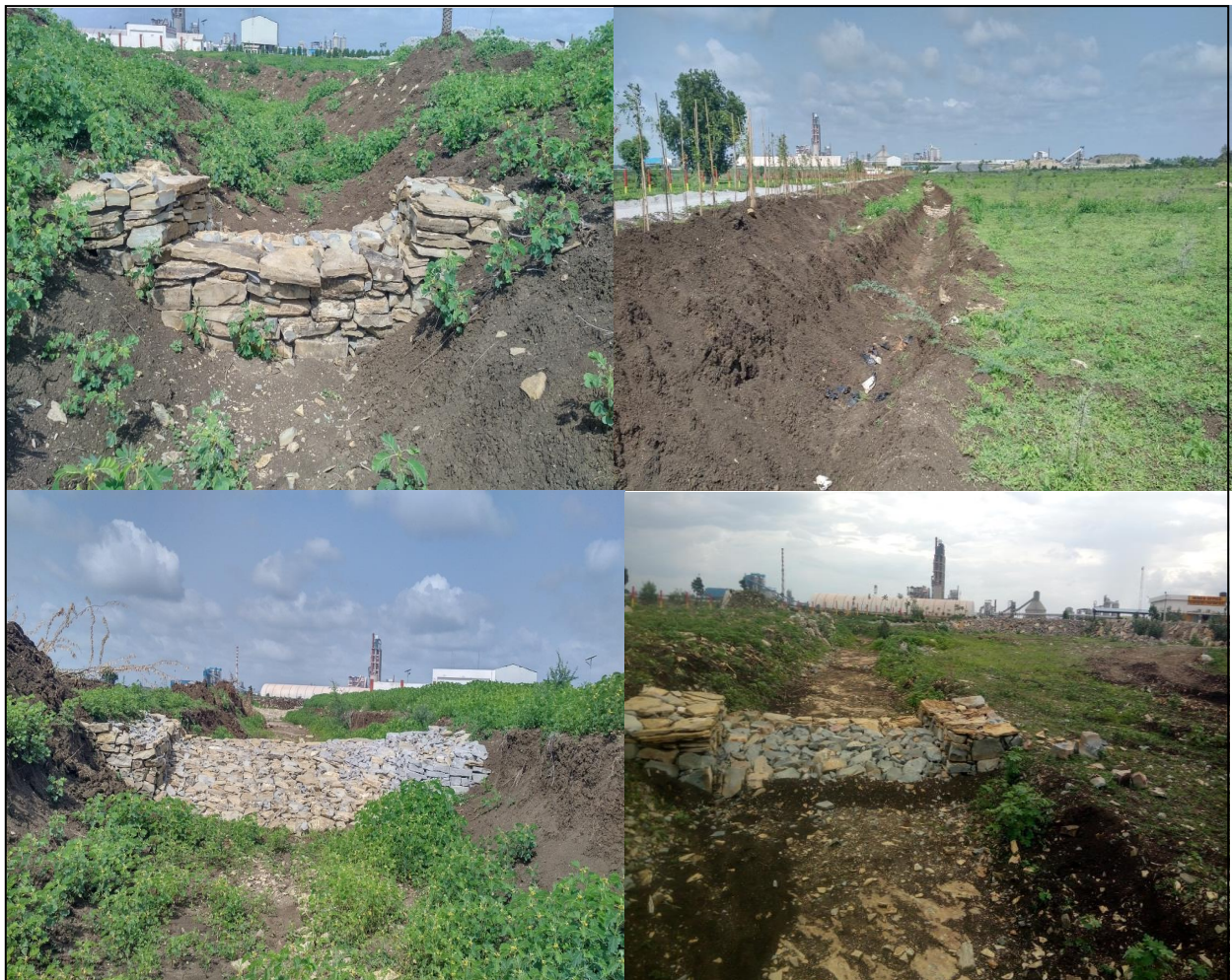
Catchment Drains with RR Dry Stone Barriers
