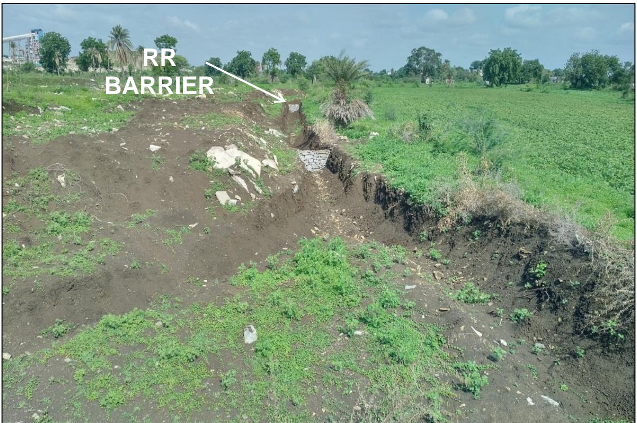
Garland drain with RR barrier
