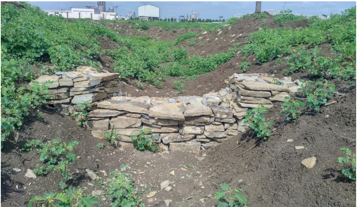
CATCHMENT/GARLAND DRAINS WITH RR DRY STONE BARRIERS
