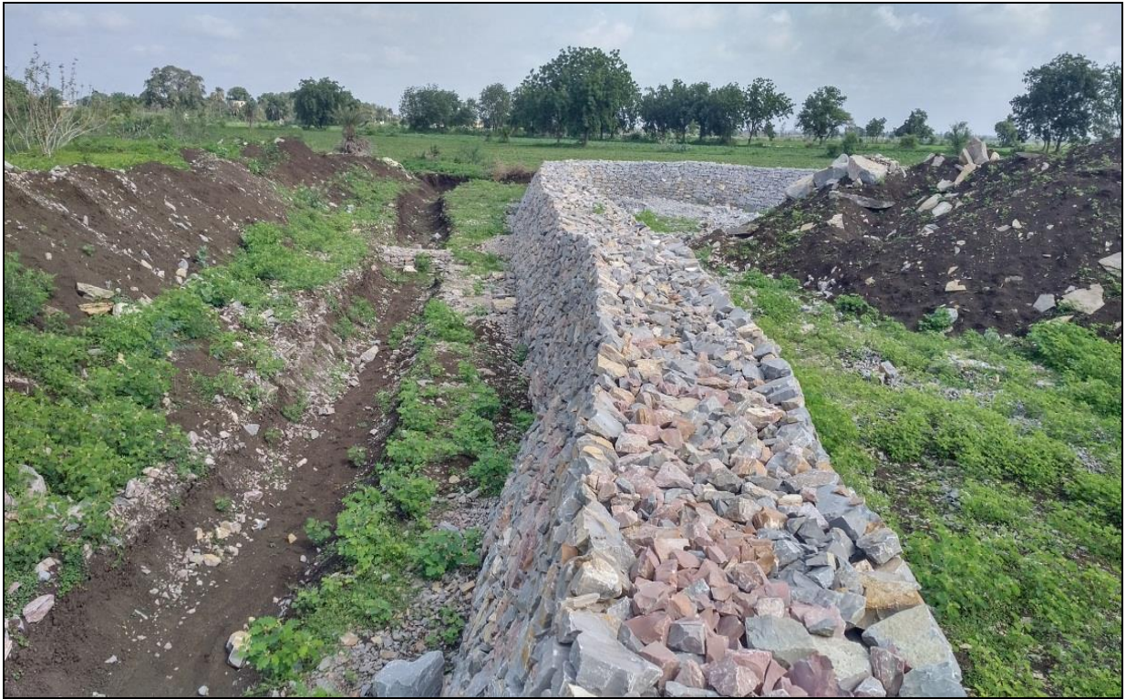
Garland Drain along the Dump Toe Wall with Random Rubble Barriers
