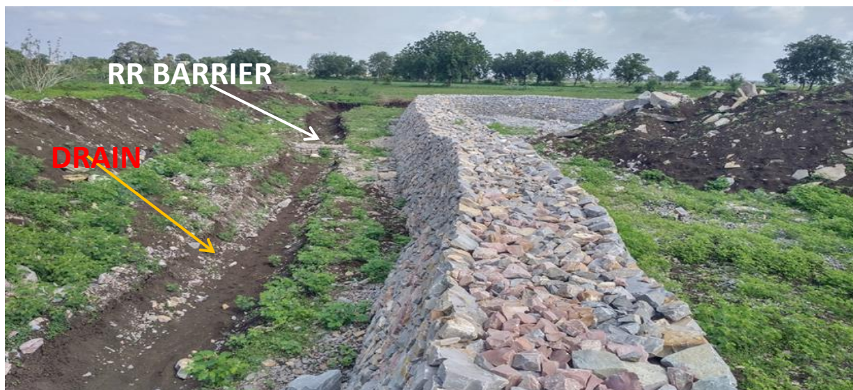
GARLAND DRAIN ALONG THE TOPSOIL DUMP TOE WALL WITH RANDOM RUBBLE BARRIERS
