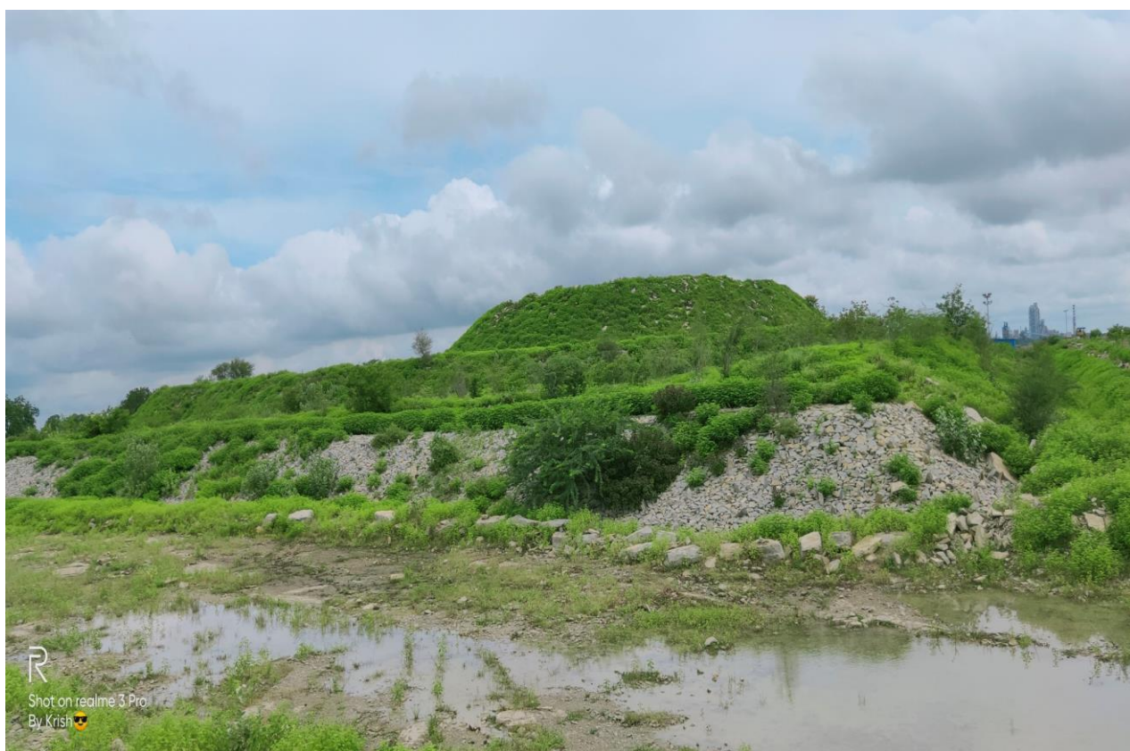
STONE PITCHING BELOW THE TOPSOIL DUMP
