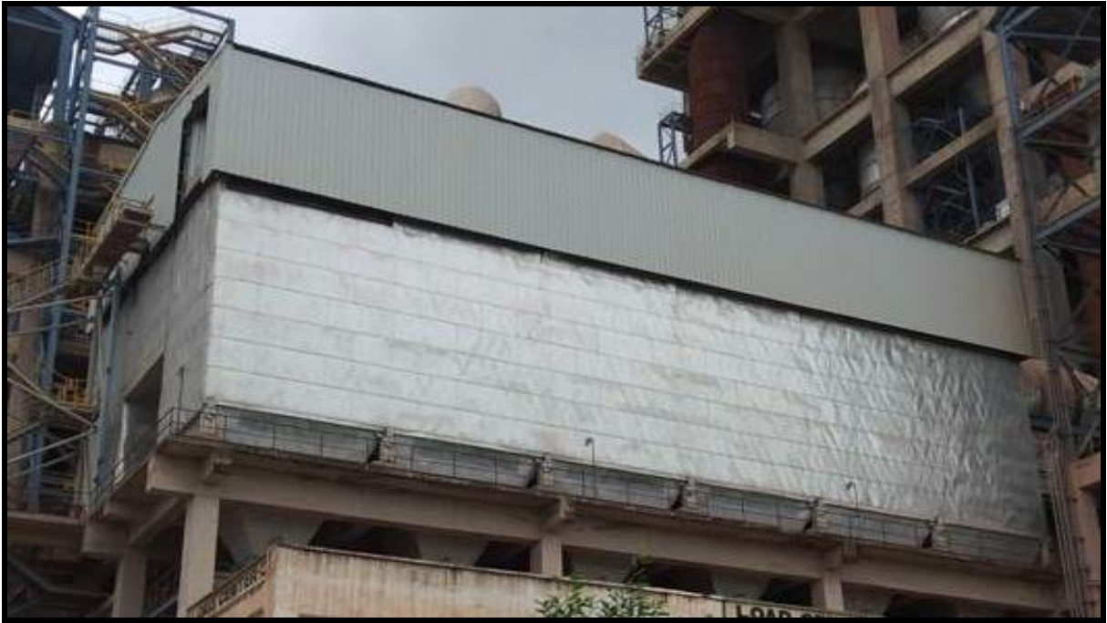
Bag House for Kiln & Raw mill
