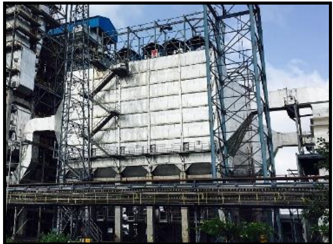
ESP for Cooler and CPP
