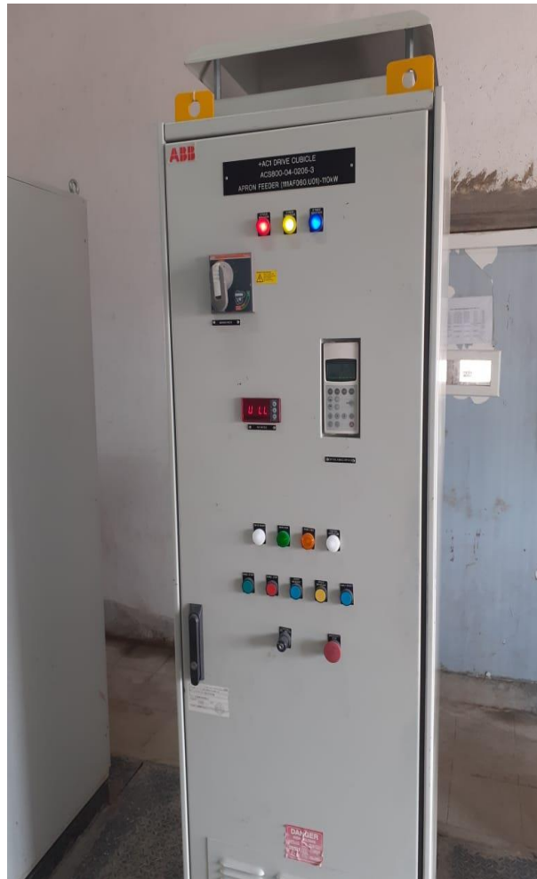
Variable Frequency Drive in 111AF060 Apron feeder
