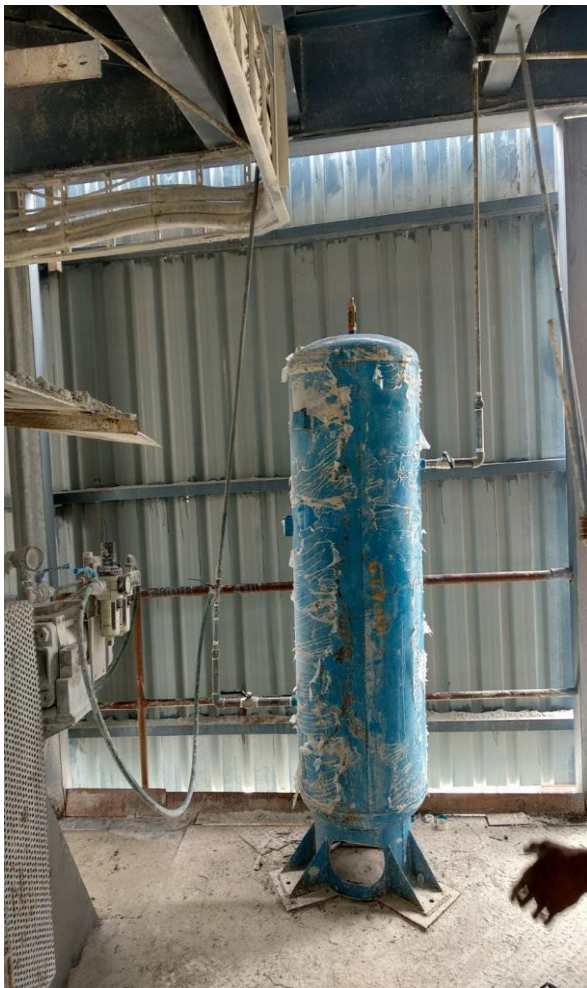
Air receiver tank with sensor at hopper to rectify air pressure drop issue
