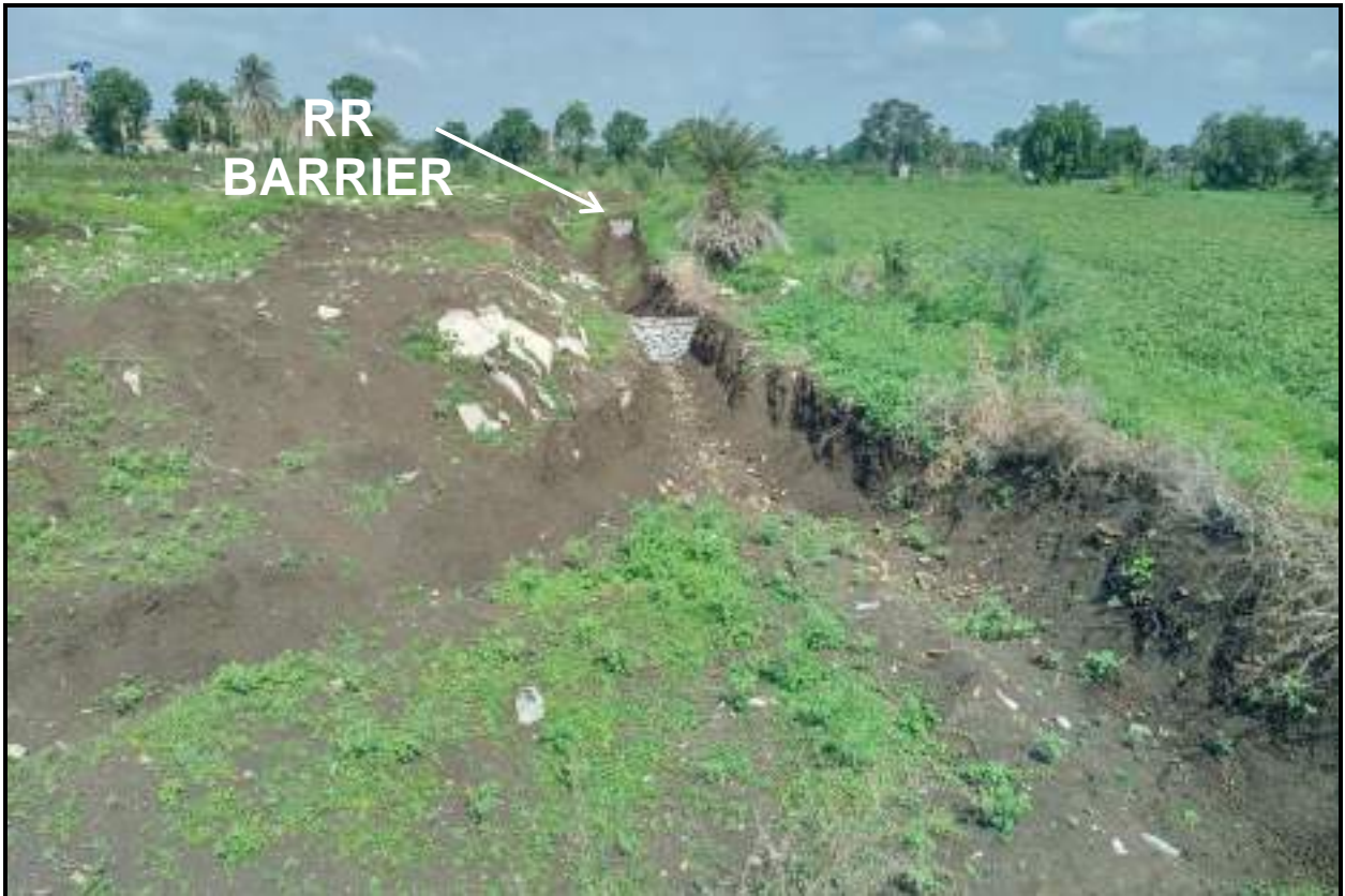
Garland drain with RR barrier
