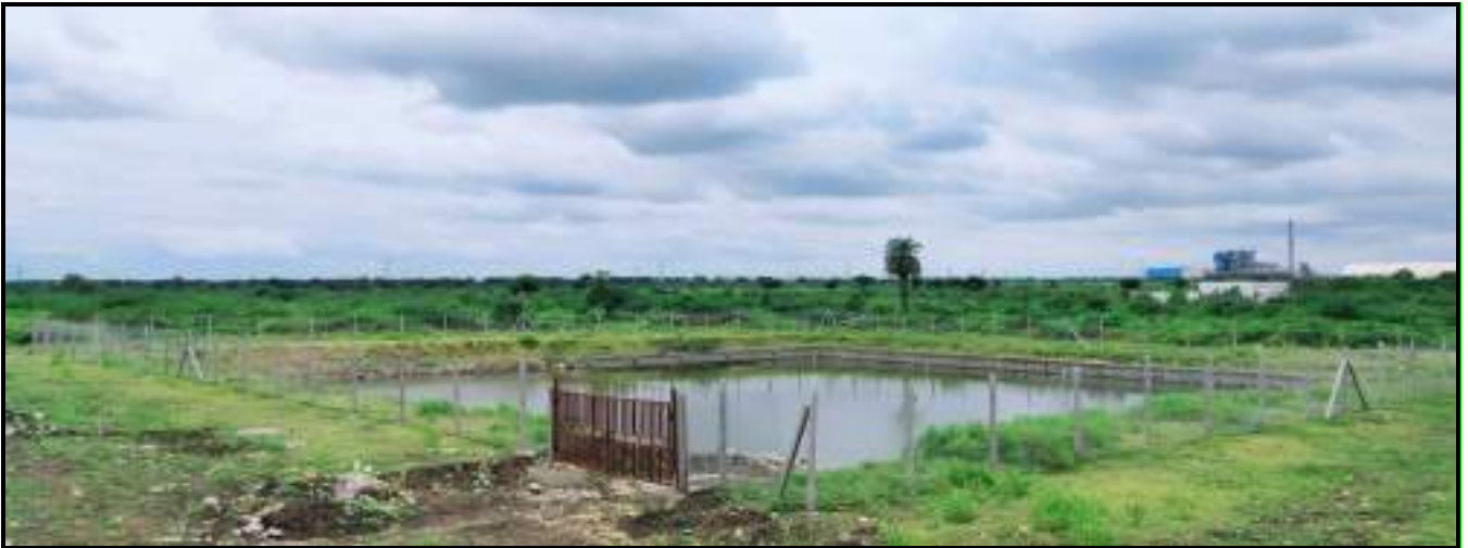
RAINWATER HARVESTING PIT cum SETTLING TANK
