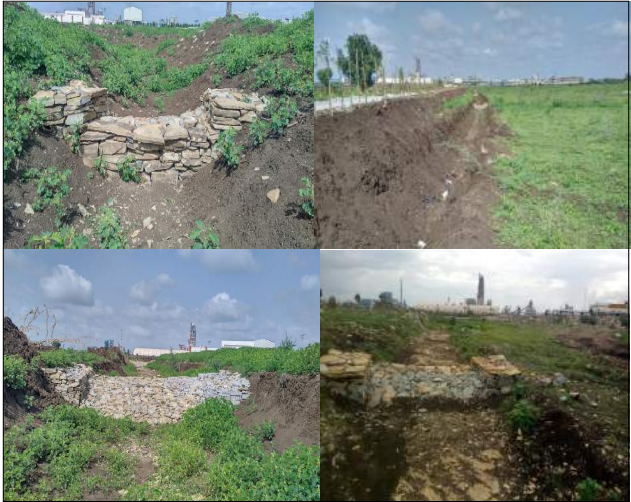
Catchment Drains with RR Dry Stone Barriers
