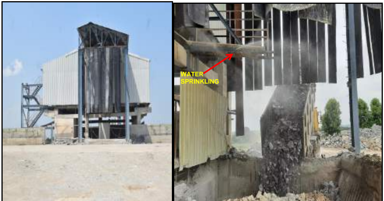
Rubber curtains & Water sprinkler system provided at Limestone dump hopper to Control dust at Lime stone Crusher
