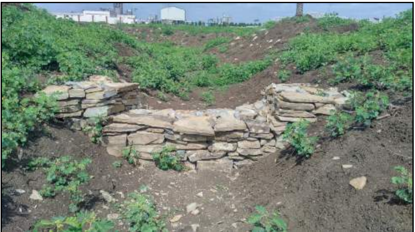
CATCHMENT/GARLAND DRAINS WITH RR DRY STONE BARRIERS
