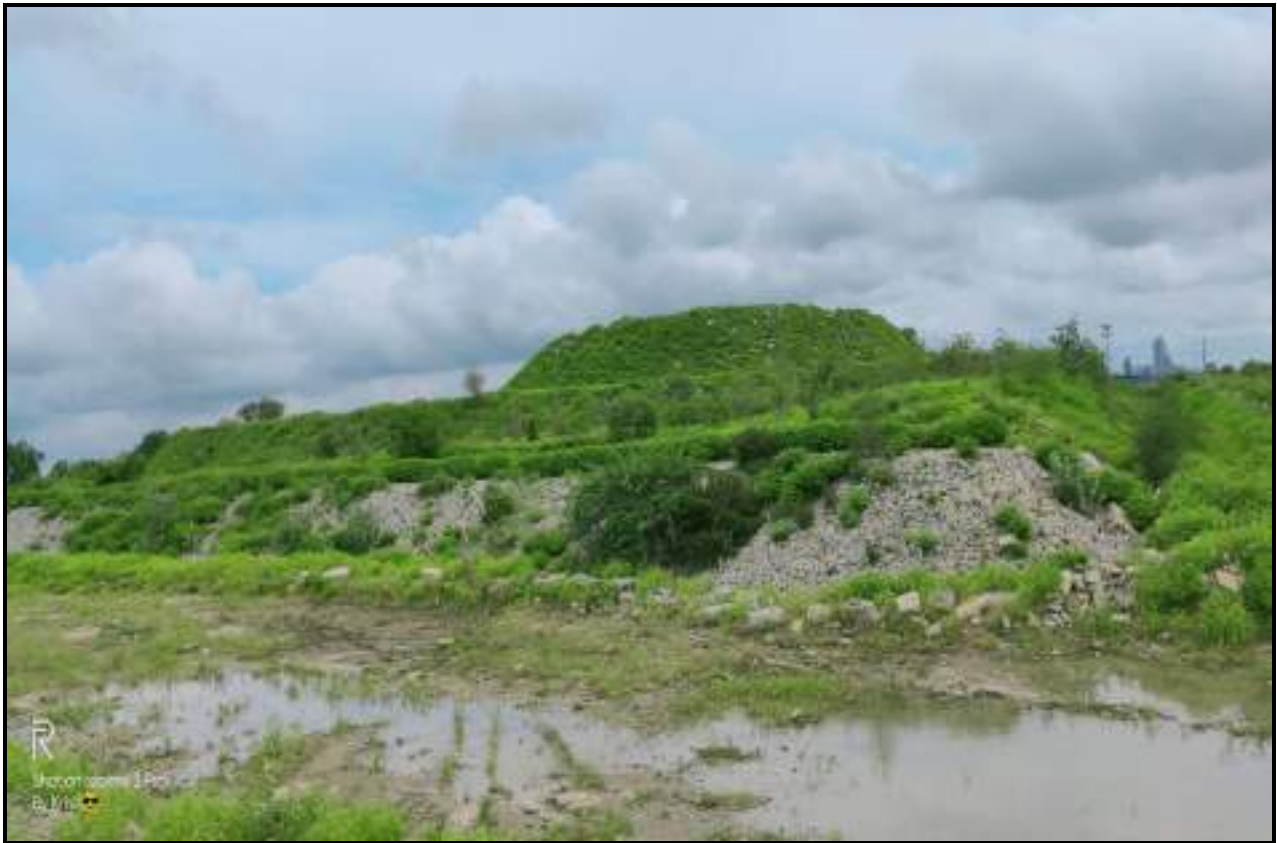
STONE PITCHING BELOW THE TOPSOIL DUMP
