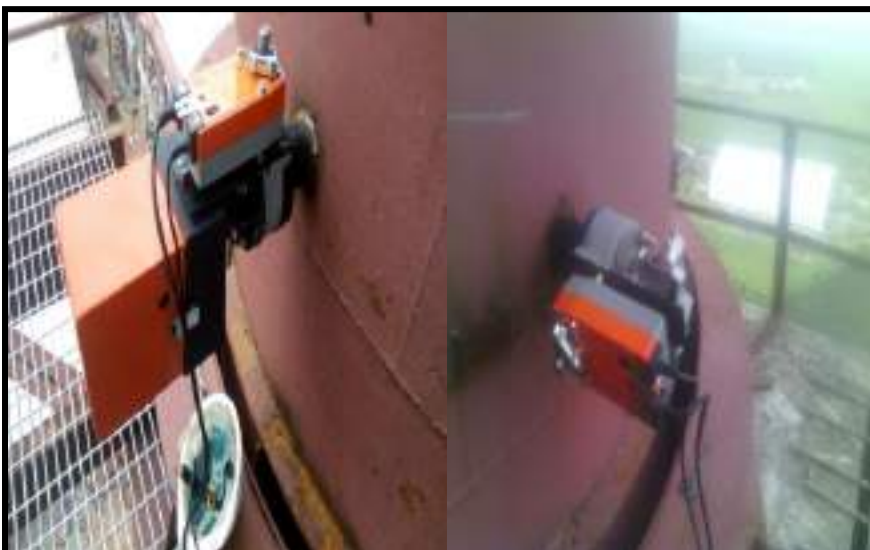
Installation of Continuous Stack emission monitoring stations for main stacks
