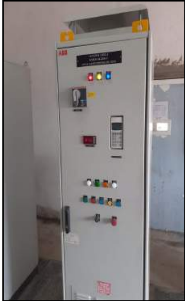
Variable Frequency Drive in 111AF060 Apron feeder
