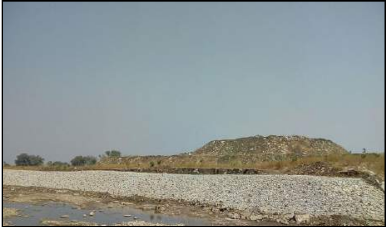
BC Soil Dump with Protection Wall
